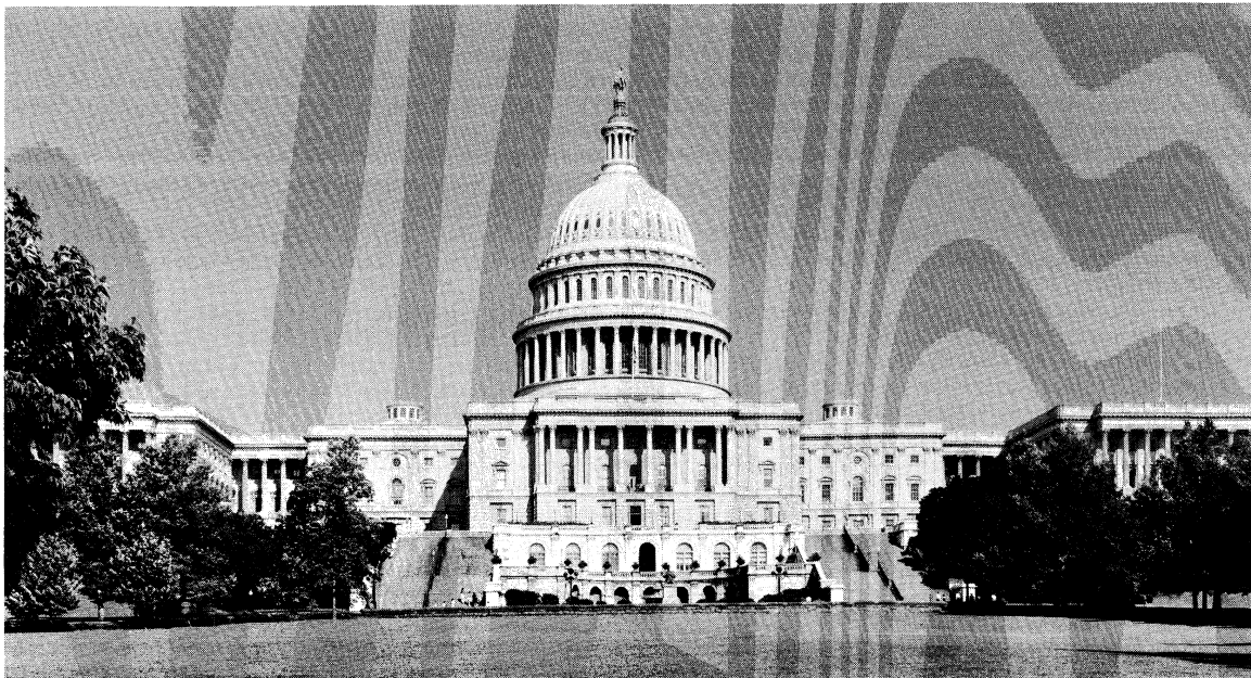
West facade with dome of cast-iron construction, U.S. Capitol building, Washington, D.C., dome begun by Thomas Ustick Walter, 1851.
