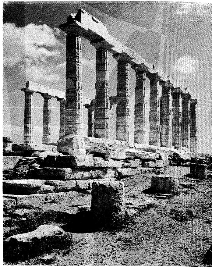
Post-and-lintel system of support, temple of Poseidon, Cape Sounion, southeast of Athens, c. 430 BC.
